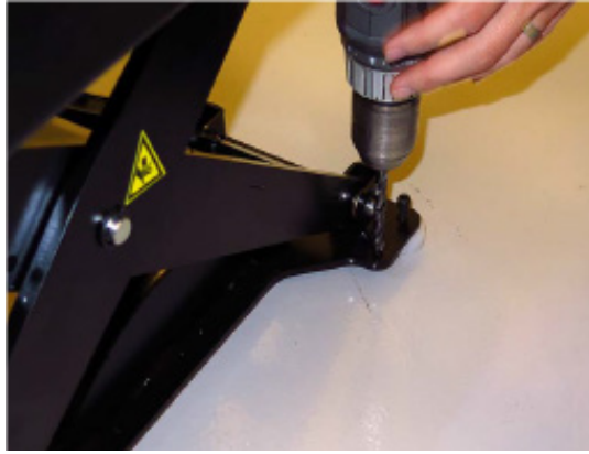
Figure 10: Use 1/4 inch masonry bit to drill the concrete
