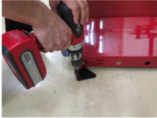
Figure 2: Drill holes - 1/4 inch bit
