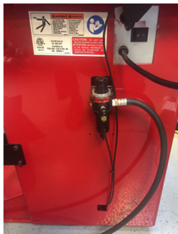
Figure 16: Air lines routed out back and zip tied
